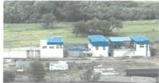
Amanora - Water Treatment Plant
