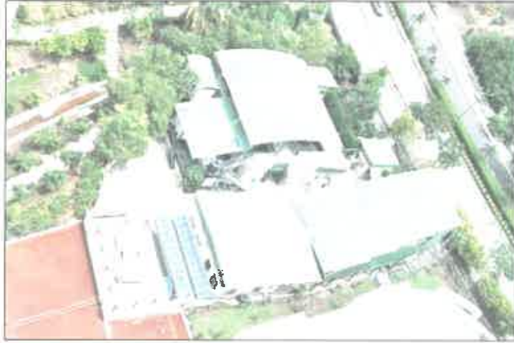
1750 CMD STP plant partially operated on Solar for first Phase of Township
